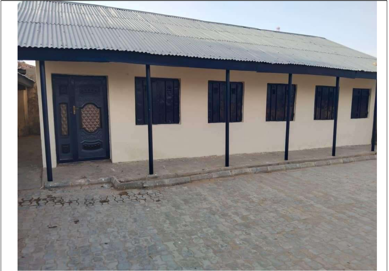
Exterior View of the ICT Building
