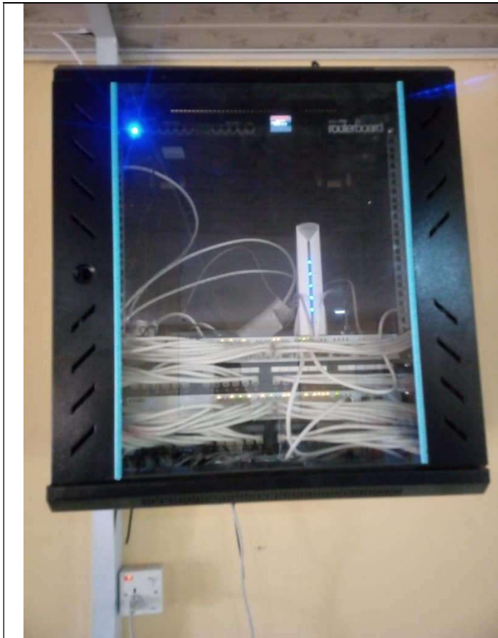
Wall-Mounted Network Rack and Administrator's Cabinet
