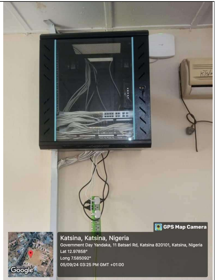
VSAT EQUIPMENT AND WALL-MOUNTED NETWORK RACK
