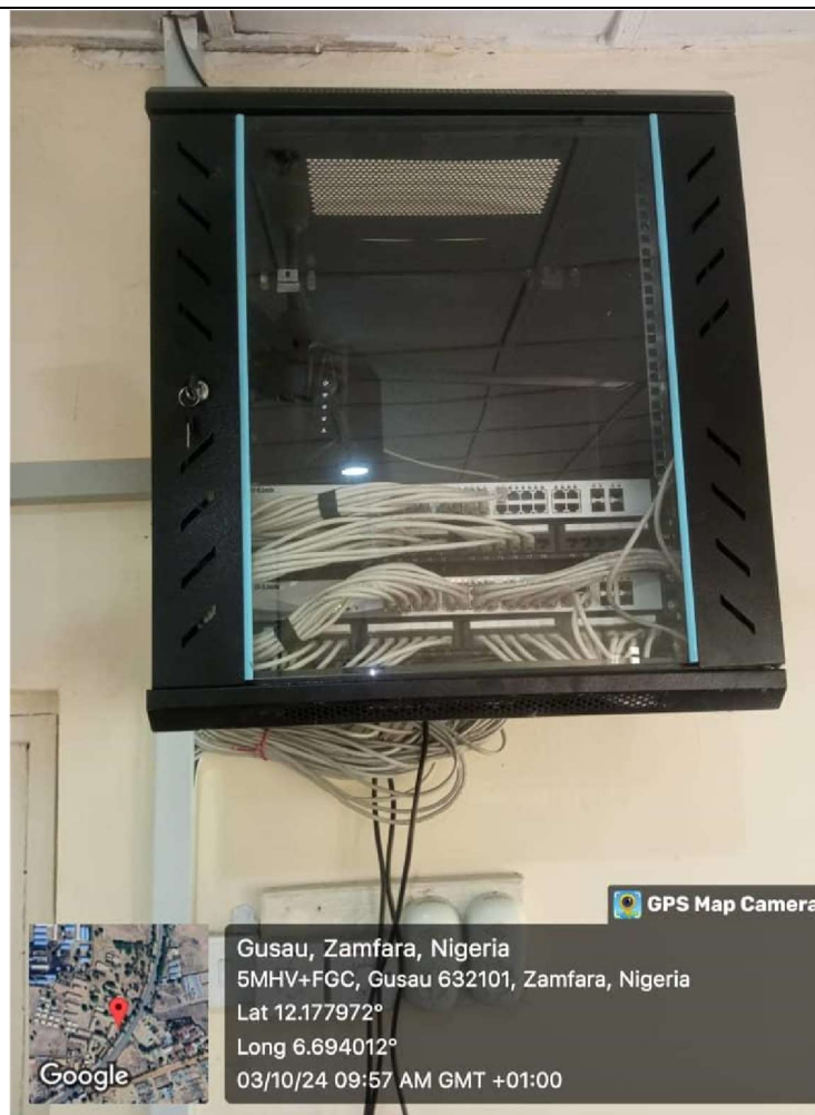
INSTALLED VSAT EQUIPMENT & WALL-MOUNTED NETWORK RACK
