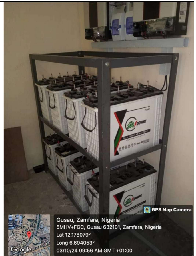
INSTALLED INVERTERS AND BATTERIES
